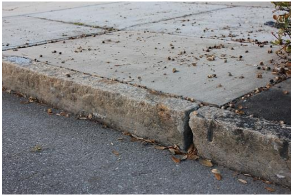
Consistent granite curbing 5 th Street North
