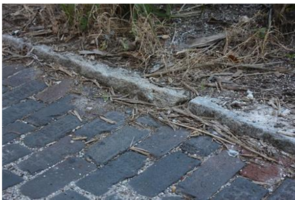
Consistent granite curbing public alley
